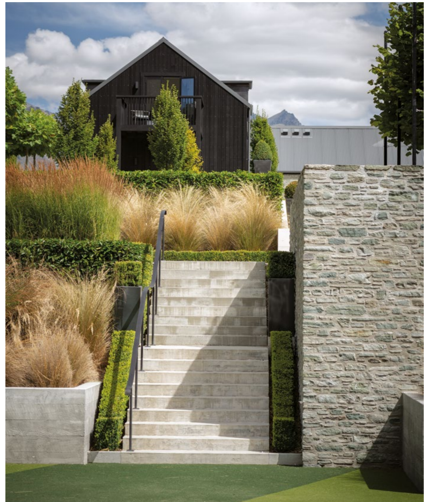
LEFT The four lime trees on the viewing platform above the tennis court will be pruned to form a square canopy when mature. ABOVE A curved powder-coated steel handrail fulfilled safety requirements as well as adding artistic interest to steep concrete steps connecting the tennis court with the higher tiers; the raised viewing platform at right sits atop a schist wall covered with a light coat of mortar for a bagged look reminiscent of early Central Otago buildings.
